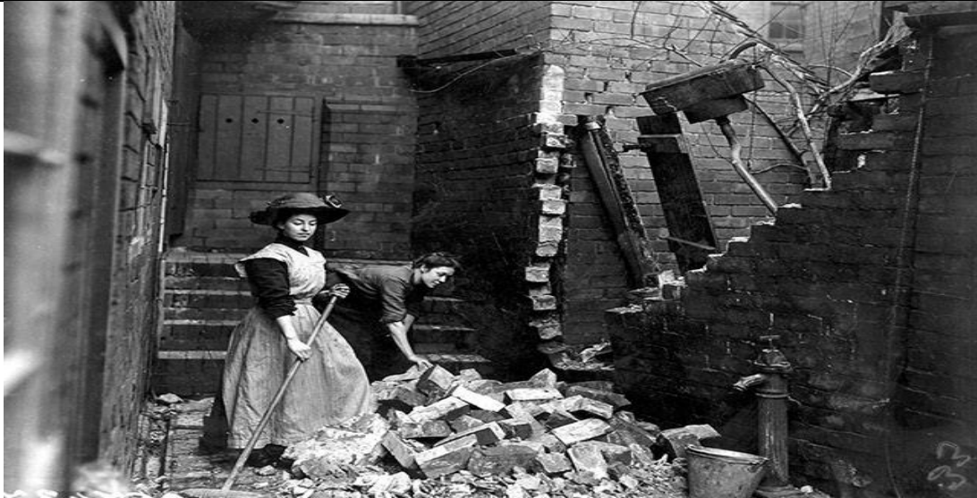
Women clearing up after the outside toilet wall and roof collapsed.
